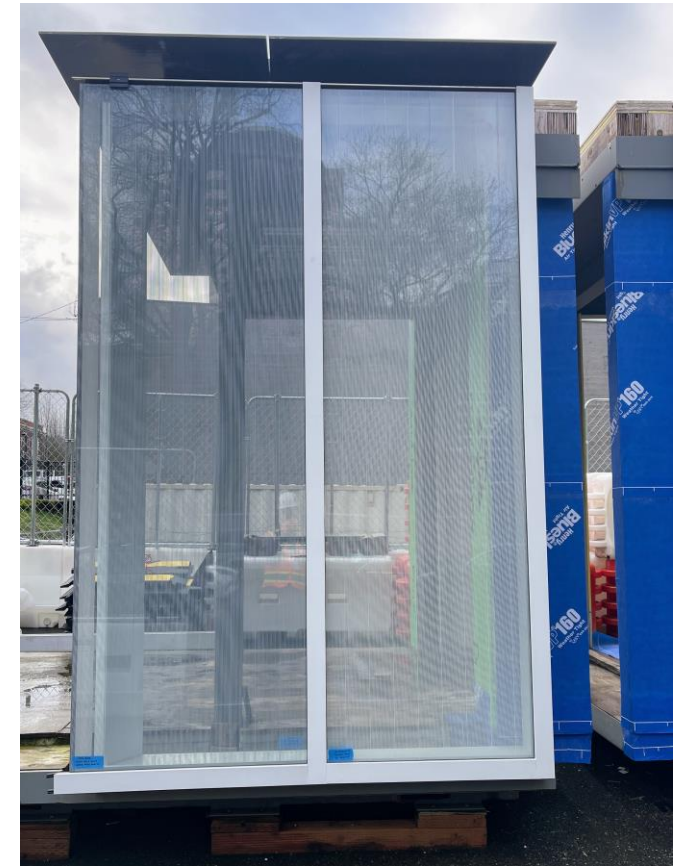
Building Mock-up – Dual and White Frit
