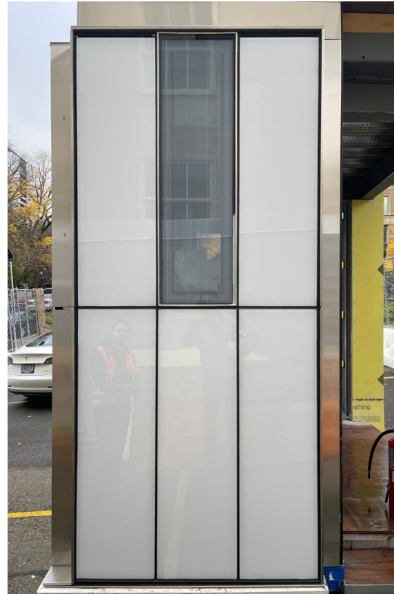
PAM - South Addition
