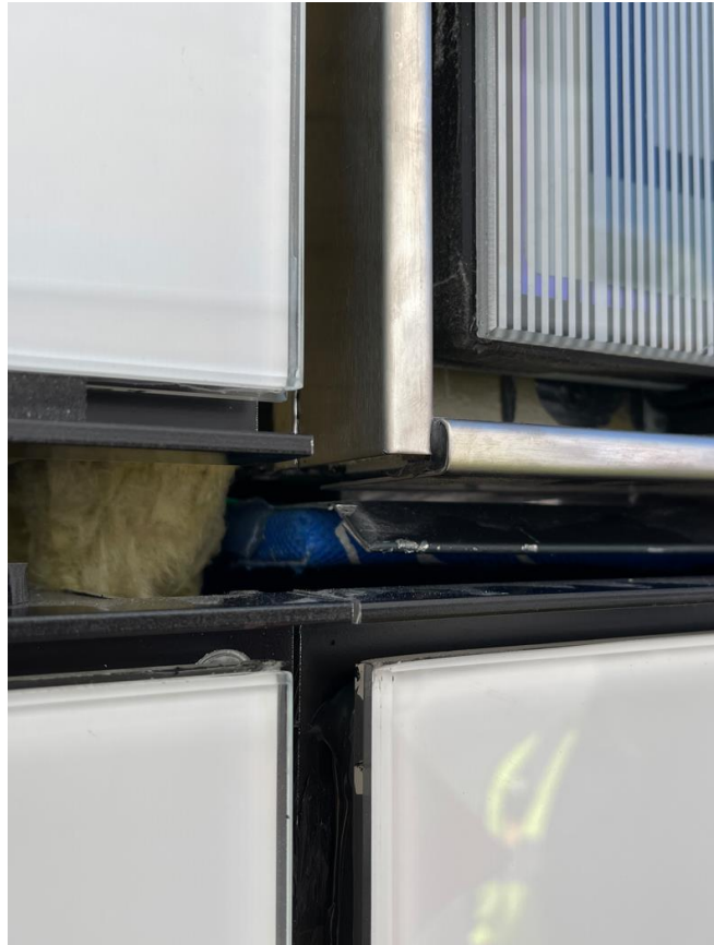
PAM - South Addition
